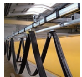
Flat cable and supports for cross travel
